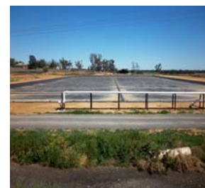
A 42ML covered anaerobic lagoon at Corowa. A 5,000 sow 'farrow to finish' piggery 2012 = 20,000 to 45,000 cows (grazing herd)
