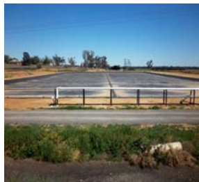
A 42ML covered anaerobic lagoon at Corowa. A 5,000 sow "farrow to finish" piggery 2012. 13,000 t/y CO 2 -e mitigated – replace LPG hot water heating
