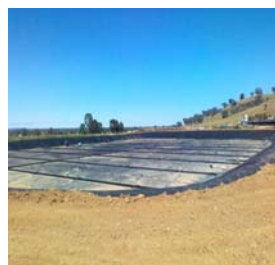
A 14ML covered anaerobic lagoon at Bungowannah. A 6,000 sow 'breeder only' piggery 2012 = 4,000 to 9,000 cows (grazing herd)
