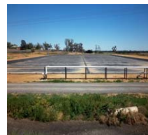
A 42ML covered anaerobic lagoon at Corowa. A 5,000 sow 'farrow to finish' piggery 2012 = 20,000 to 45,000 cows (grazing herd) = 3,500 to 6,000 cows (freestall)
